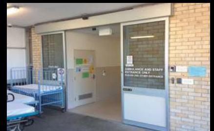
Monavale Hospital Ambulance Bay. Installed DSL 125 System.
