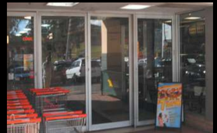
Parkside Plaza, Miranda. Talbot replaced the old system with new.
